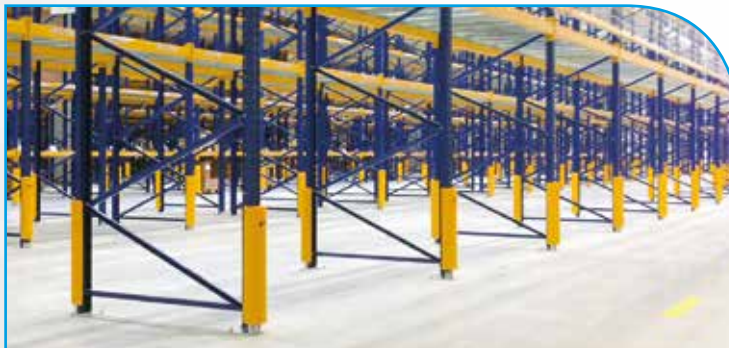
Schneider Electronics new warehouse full installation - (France).
